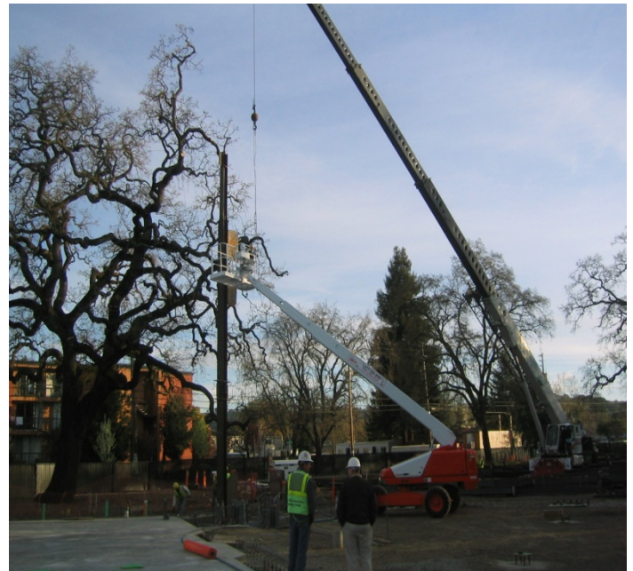
Above: Single crane and crew used during erection process
